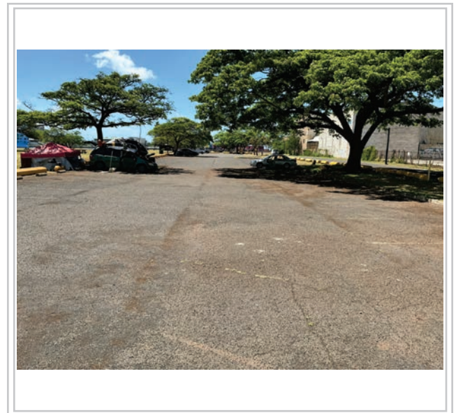
Area to be repaved
