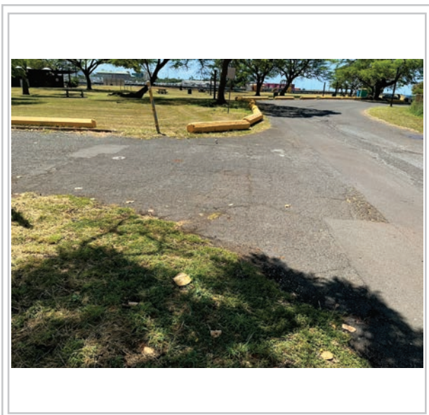
Area to be repaved
